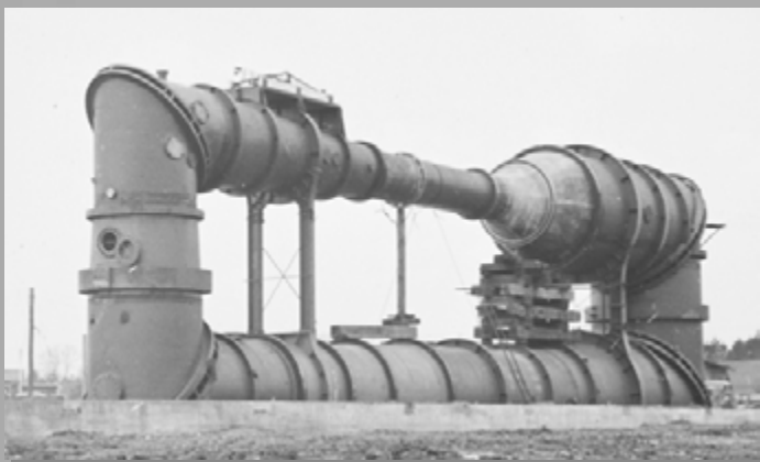
Construction of the Garfield Thomas Water Tunnel - 1949
